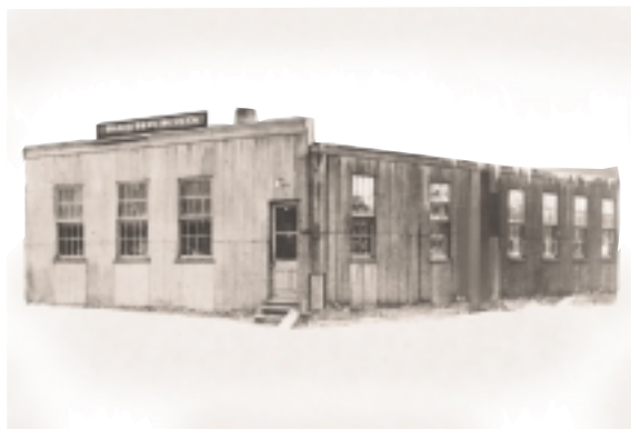
Original 1902 Mendota Plant
